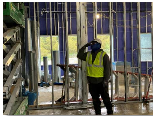
Students receive hands on electrical training.
